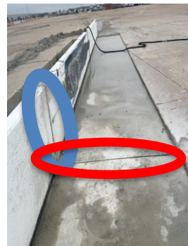
Fig 4: The Test Bridge
