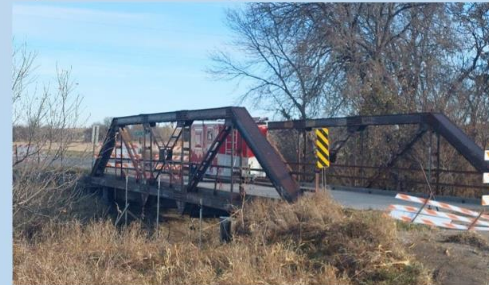
Tested truss bridge
