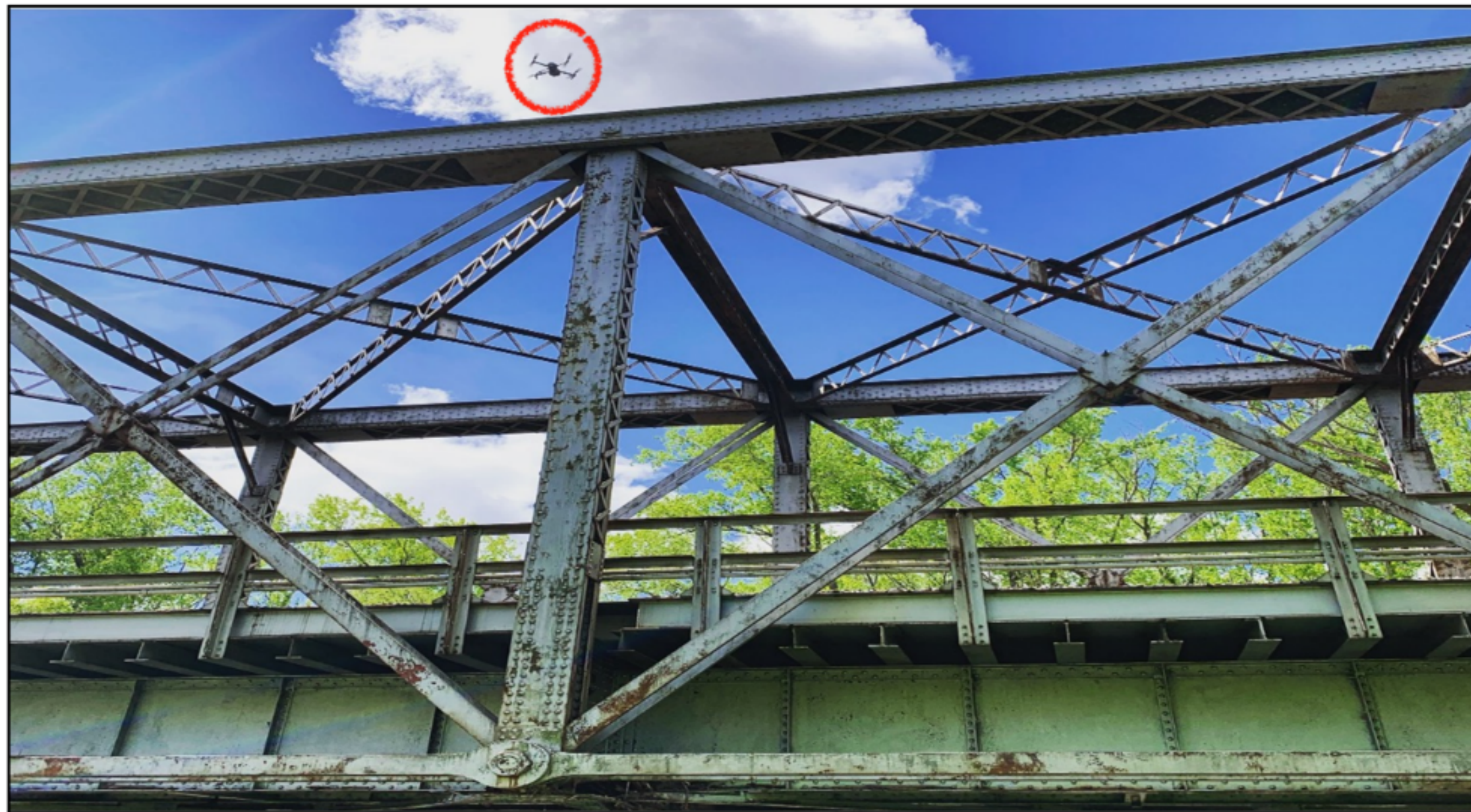
Steel bridge inspection using UAVs
