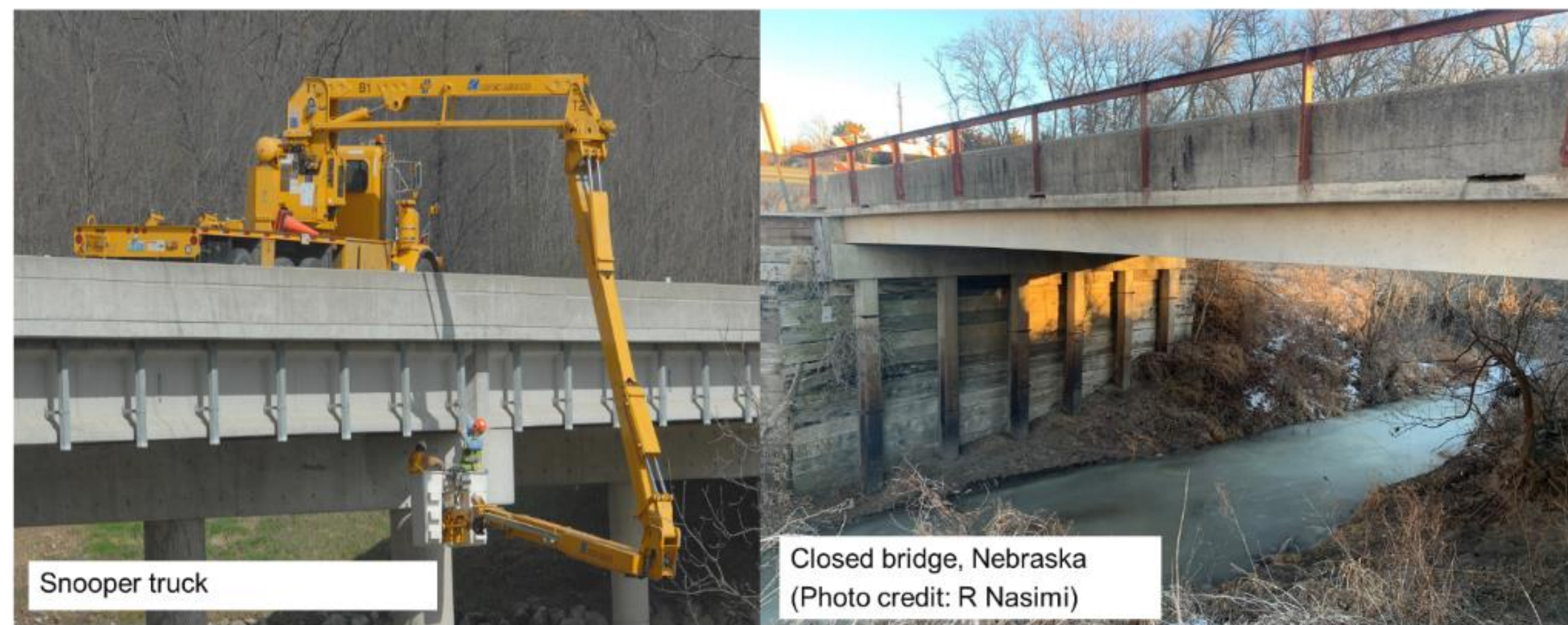
Traditional Bridge Inspections
