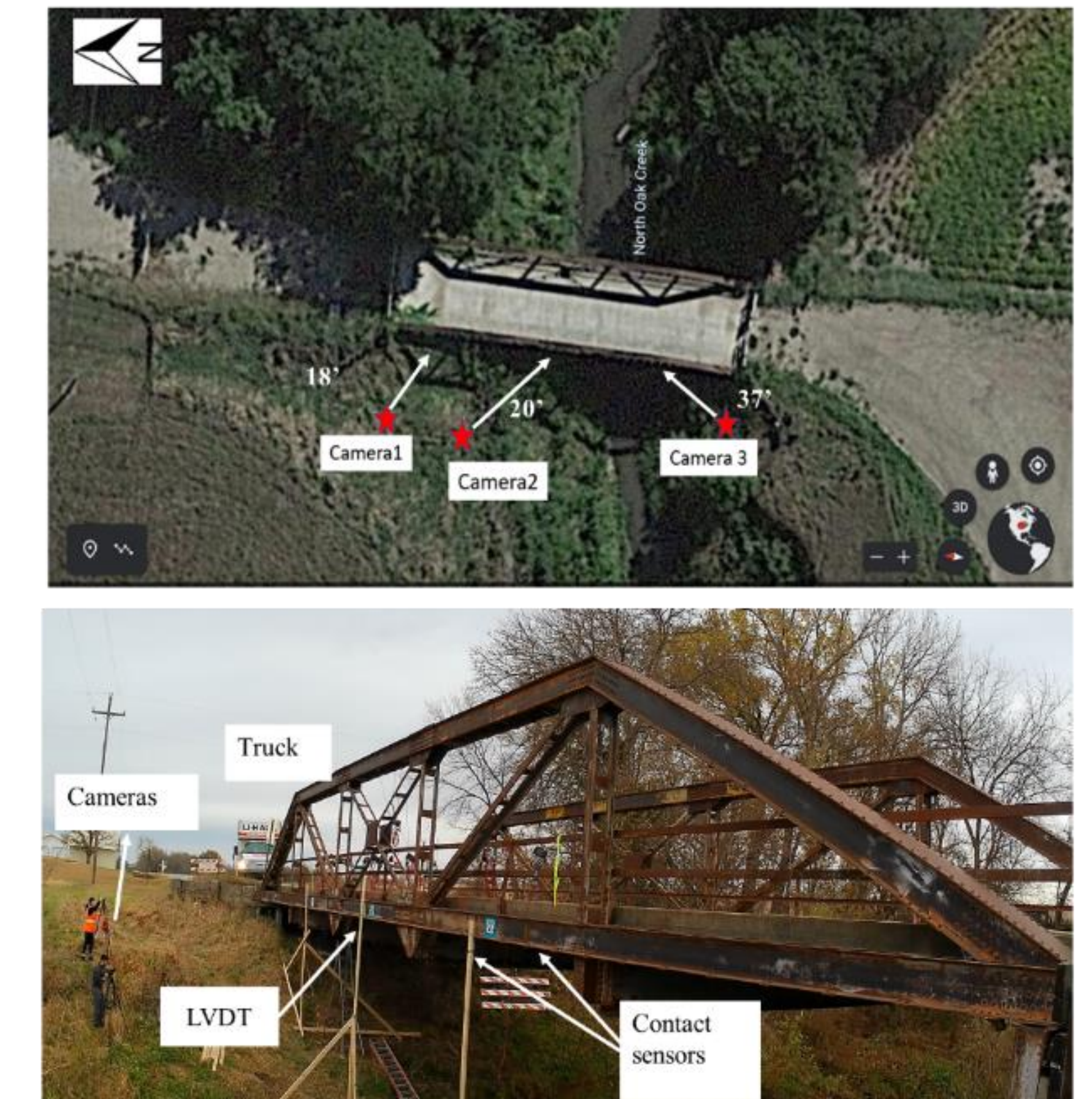
Bridge instrumentation and experiment
